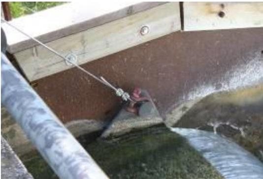
To make a dam adjustment, one WLC member cranks the winch wheel while another WLC member measures the vertical distance between the gate and a reference point on the side of the dam. A specially calibrated “yard stick”, complete with a leveling bubble, is used to make sure the measurements are accurate. Eight rotations of the winch wheel results in about one inch of vertical movement of the gates, which
